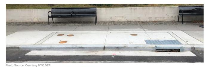
Figure 9: Example of Concrete Top Infiltration Basin
