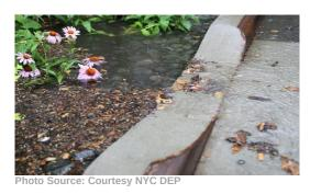
Figure 1: Cut for stormwater conveyance
